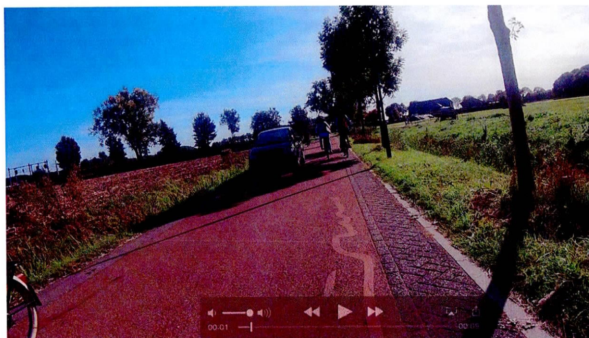
Figure 4 Example of optical narrowing of a road. The different colour bricks encourage everyone into the middle of the road, which tends to slow all traffic down.
